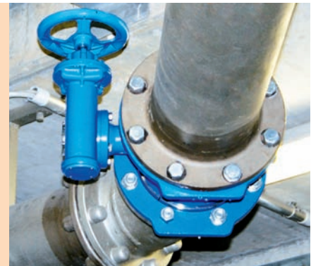
Figure 3 - Perfect fit of the valve ensures top operability in all installation situations. It is even possible to subsequently turn the valve when it is installed.
