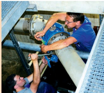
Figure 2 - Valve replacement is facilitated by pulling up the loose flange - spreading the valve flange and pipe flange to enable installation of the seal is no longer necessary.
