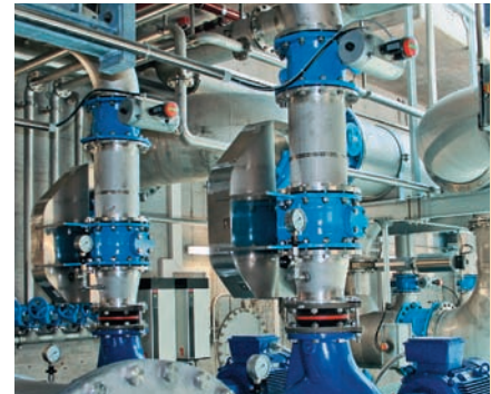
Easy installation in vertical pipes. No time-consuming bolstoring of the valve during assembly, as the valve is fastened to the fixed flange during installation.
